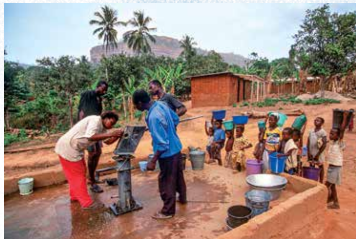
Rose Akyemah and other Asikam village volunteers repair one of three well pumps World Vision installed in 1991.
